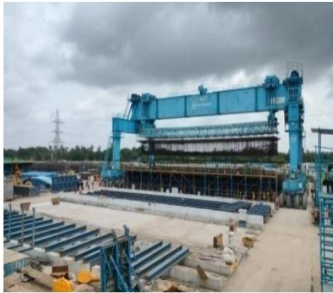
Fig 7: Straddle Carrier lifting steel cage, at stacking yard
