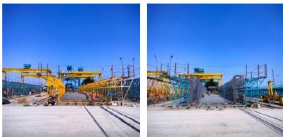
Fig 9: Rebar tying in Jig
