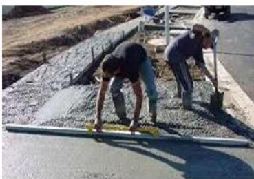
Fig 23: Manual Hand Screeding
