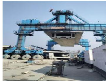
Fig 39: Double Stacking of FSBG Span
