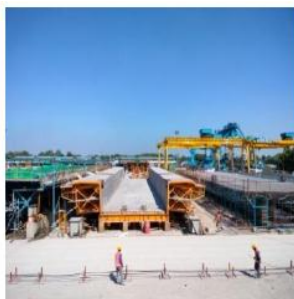
Fig 14: Outer Forms with Soffit
