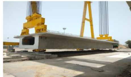
Fig 4: Full Span Box Girder at Stacking Yard
