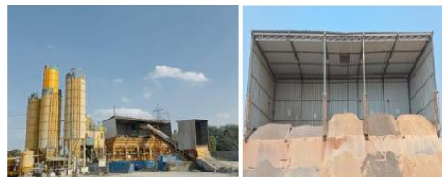
Fig 26: Batching plant bins of aggregate are covered with GI sheets to maintain temperature
