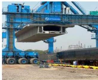
Fig 38: Straddle Carrier Shifting of FSBG
