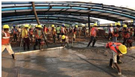
Fig 3: Casting of Full Span Box Girder -top slab
