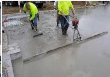
Fig 24: Vibrating Screed
