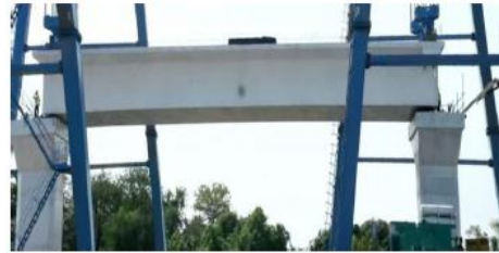
Fig 2: Casting of Full Span Box Girder
