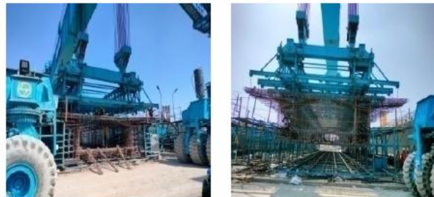
Fig 10: Straddle carrier lifting Rebar cage from Jig
