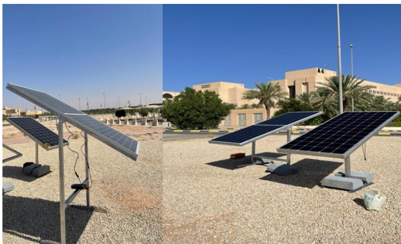
Figure 1. Installation of the bifacial module at different elevations
