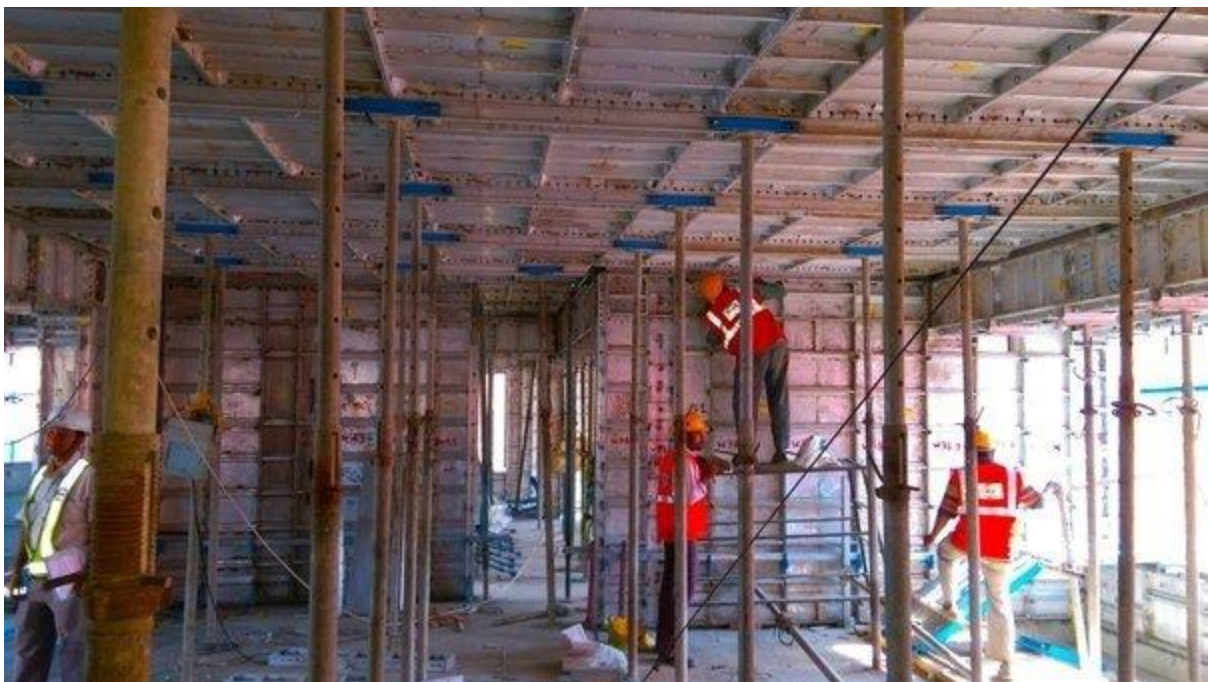
Fig.3. Horizontal formwork systems used to form the horizontal concrete work slabs or roofs.
