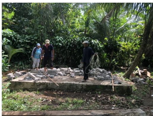
a. Brick Foundation Work
