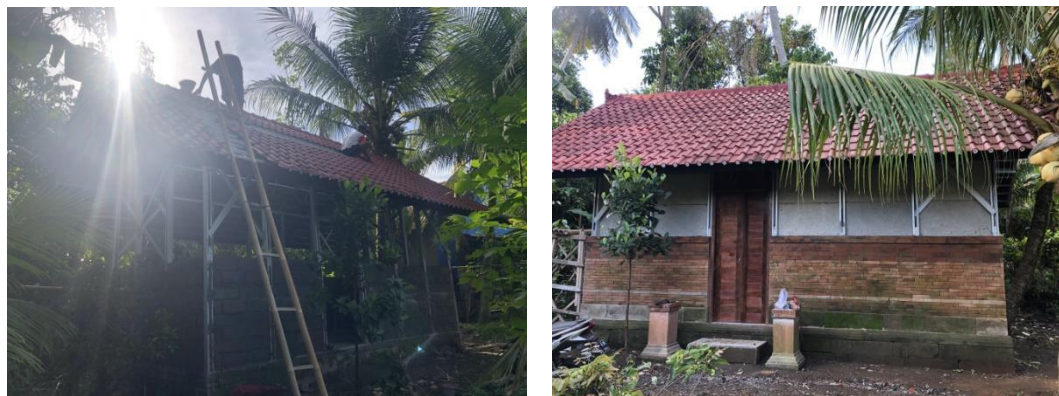
a. Roof installation work b. Finish House (Physical 100%)
