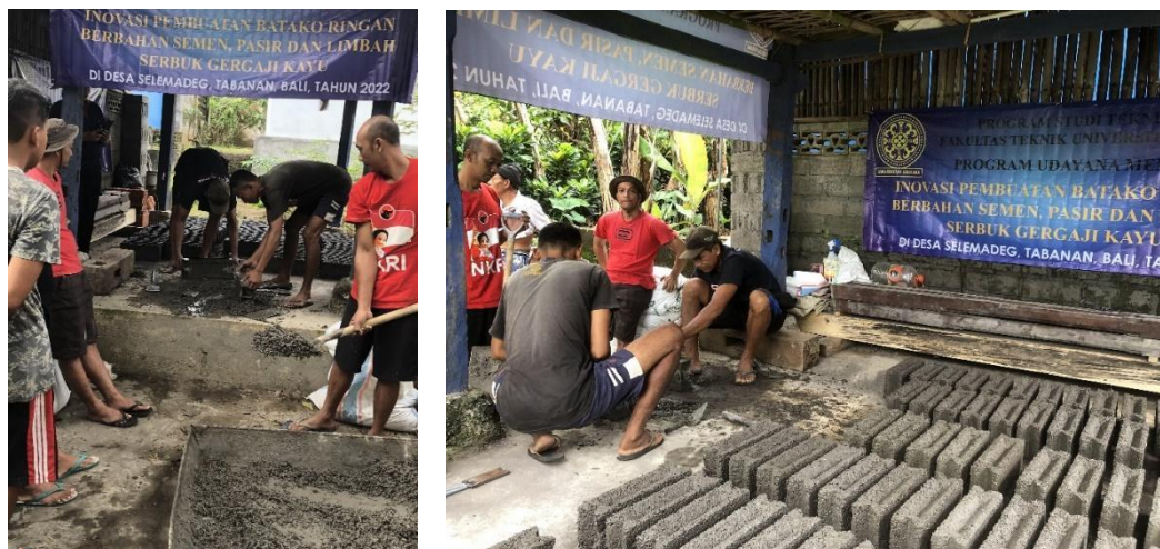
Figure 3, Process and Results of Manufacturing Panels and Local Sawdust Bricks
