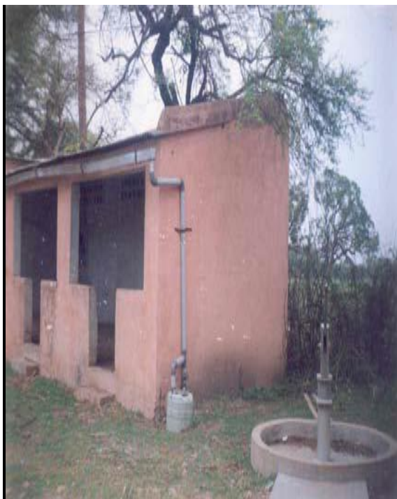
Figure 3: Roof Top Harvesting, Injection Well
