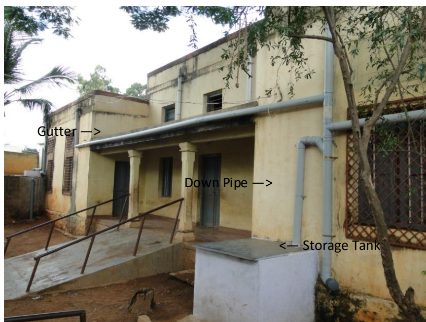
Fig-3 : Rooftop rainwater harvesting in a school building.
