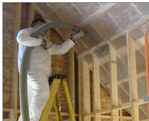
FIG.3. BLOWING CELLULOSE IN TO RAFTER BAYS.
