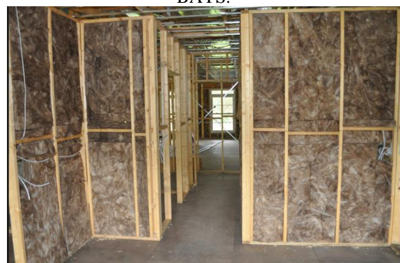
FIG.4. EARTHWOOL BULK INSULATION INSTALLED ON WALLS.
