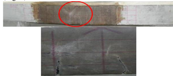
Figure 7a: Flexural Failure and Rupture of Fabric of Beam A1Y
