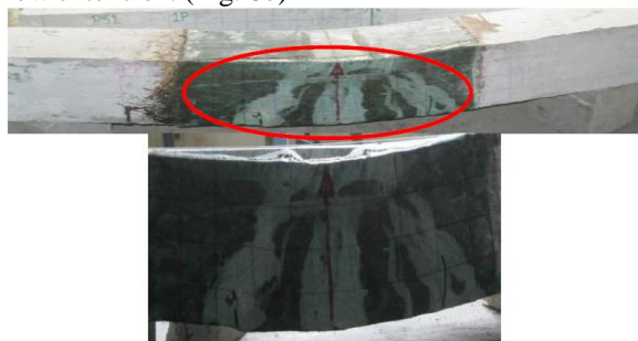
Figure 9a: Flexural Failure and Debonding of Fabric of Beam C1Y
