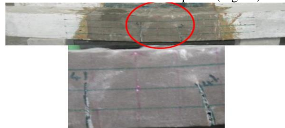
Figure 7b: Flexural Failure and Rupture of Fabric of Beam A2Y
