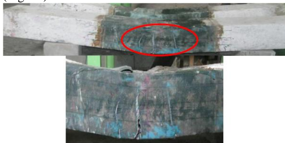
Figure 8b: Flexural Failure and Rupture of Fabric of Beam B2Y
