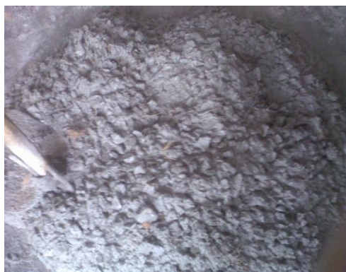
Figure-1: Mixing of Aggregates
