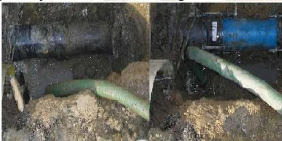
Figure 2.5 mains repaired connection at sector 21
