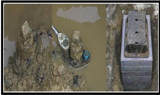
Figure 2.4 sluice valve repair
