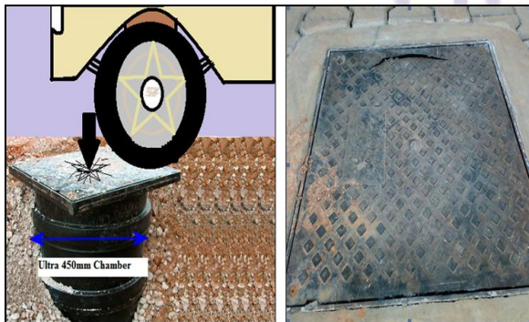
Fig no.03 Broken of the uPVC cover plate under load exerting by vehicle when it passes.
