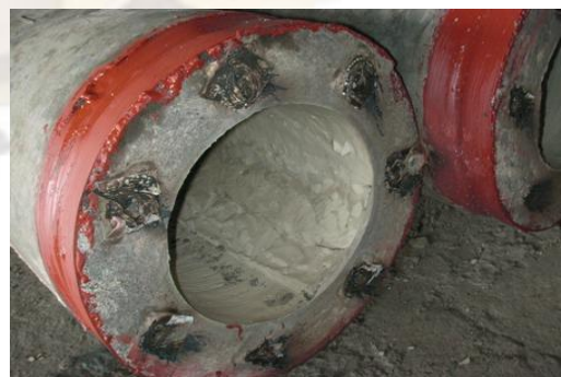
Figure 1 Roughly internal surface of hollow-core concrete pile
