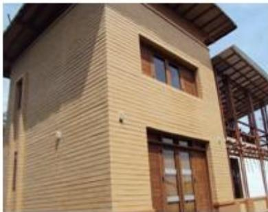
Picture 5. Housing built with SCB.
