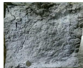
Figure 20 Broken Structure of Brick
