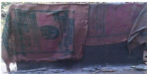
**Fig. 3 Curing of beam**
