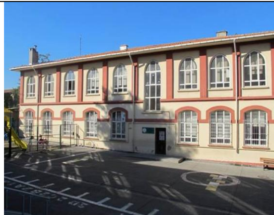
Figure 6. Fatih Counseling And Research Center (Former Vezneciler School For Impaired Hearing)
