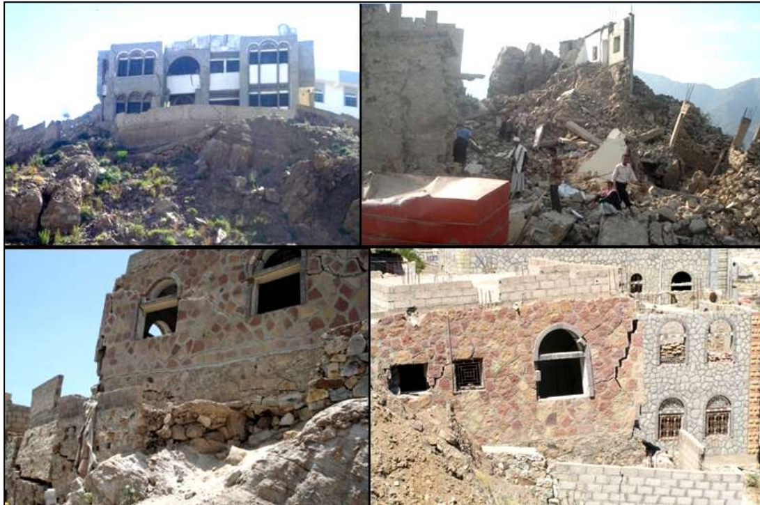
Fig.1 Photographs showing dilapidated conditions of buildings underlain by Tertiary volcaniclastics in the study area [4]
