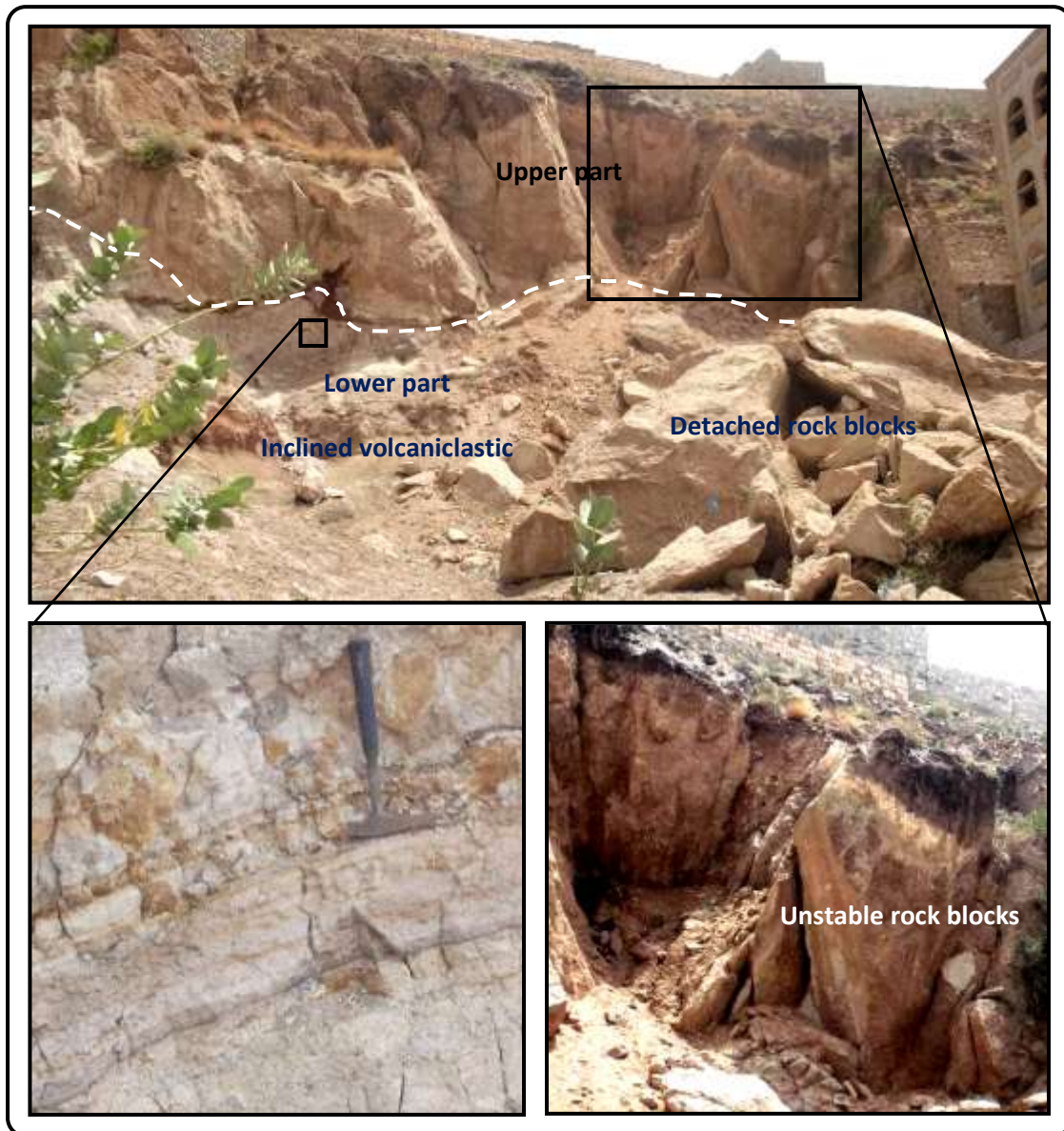
Fig. 7 Field photograph of the slope of station No.30 (zone-I) showing two different lithologies of the slope. Note the unstable columnar blocks in the upper part as well as the detached rhyolitic tuff blocks settled at the toe of the slope
