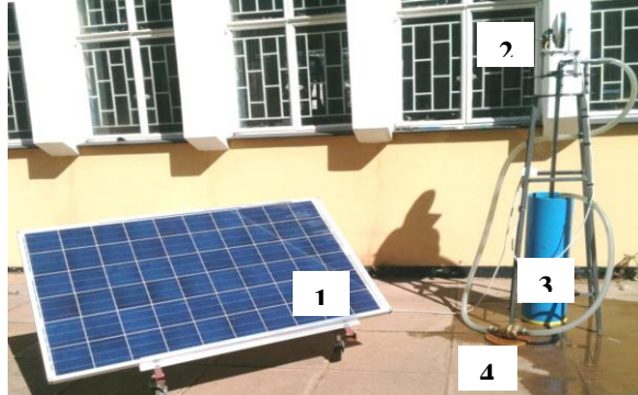
Fig. 3 Side view of the solar powered sonic pump where: 1- solar panel 230W-80V, 2 – shaker and the spring system, 3- the well, 4 – the water meter type C-PHB 3122 of 2.5 m 3 /h metering capacity.
