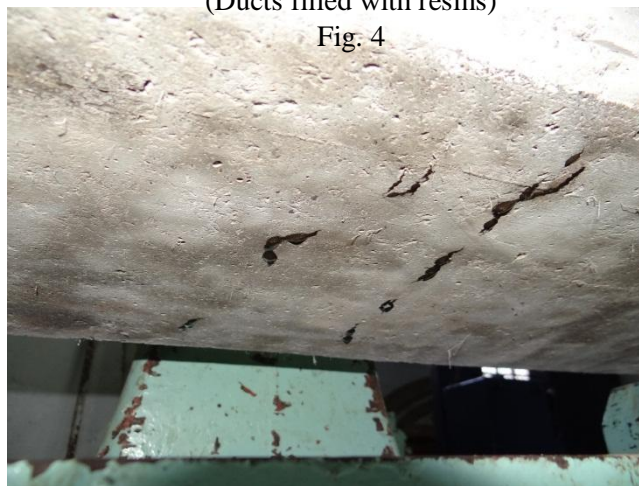
Soffit of slab after loading and crack formation Resin is released from voids through cracks
