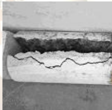
Fig. 4 View of Failed Cylinder RS00
