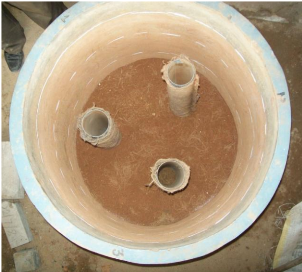
Fig.6a Installation of vertical drains
